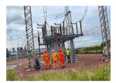
ECNEL, jointly with the EPC Contractor and EDM, successfully erected the Civil foundations for the new CSE cable sealings, all the Electrical parts until the energization of the new 66kV composite outdoor terminations.
